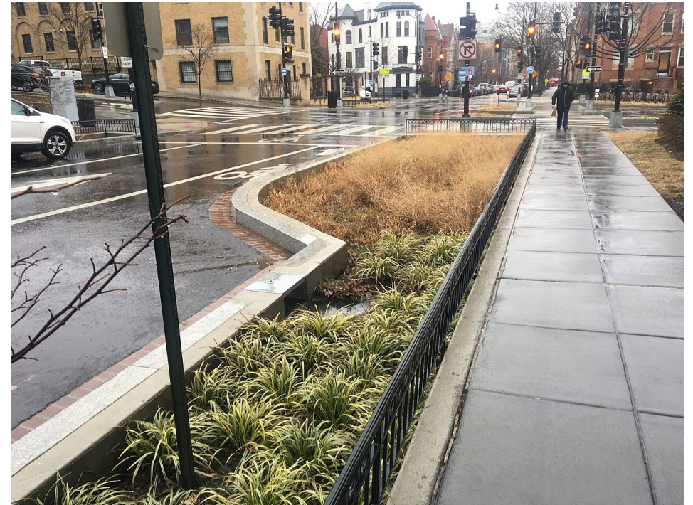
Example of an urban bioswale used to collect stormwater
