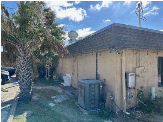
East side of the clubhouse
