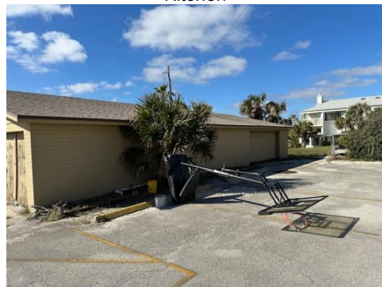
East side of the garage
