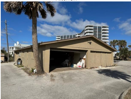
South side of the garage
