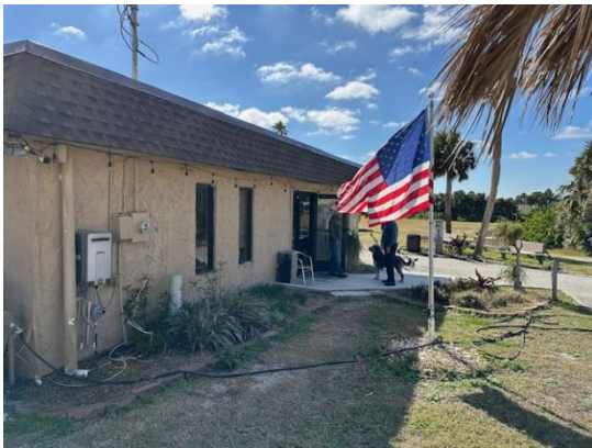
North side of the subject clubhouse
