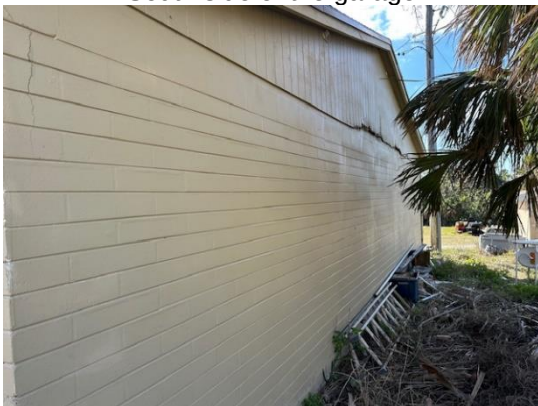
North side of the garage
