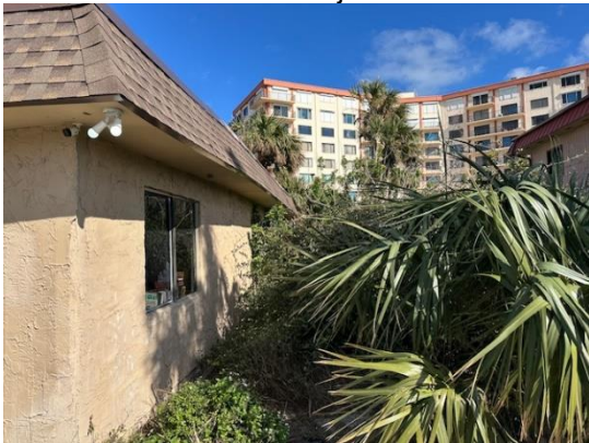
South side of the clubhouse
